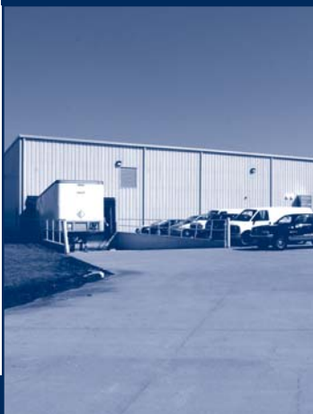
Current Records Center, 3765 Winchester Rd.
